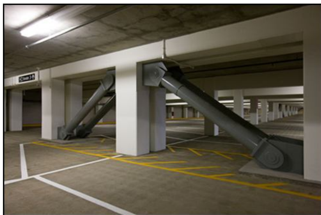
Construction of John Wayne Airport Parking Structure
